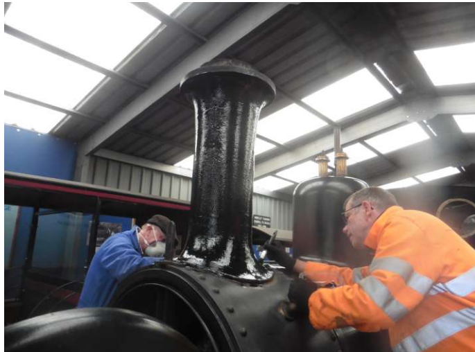
I wire-woolled and cleaned the sliding bars, and the smokebox door handles
